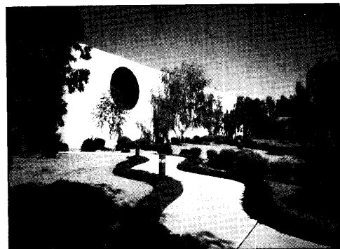
Tempe, Arizona: New 170,000-square-foot wafer fabrication facility.
